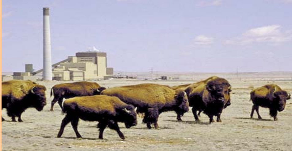
4. Home on the range. The Rawhide Energy Station must be the only power plant in the U.S. that maintains a herd of award-winning American bison on surrounding plant property. Courtesy: Platte River Power Authority
